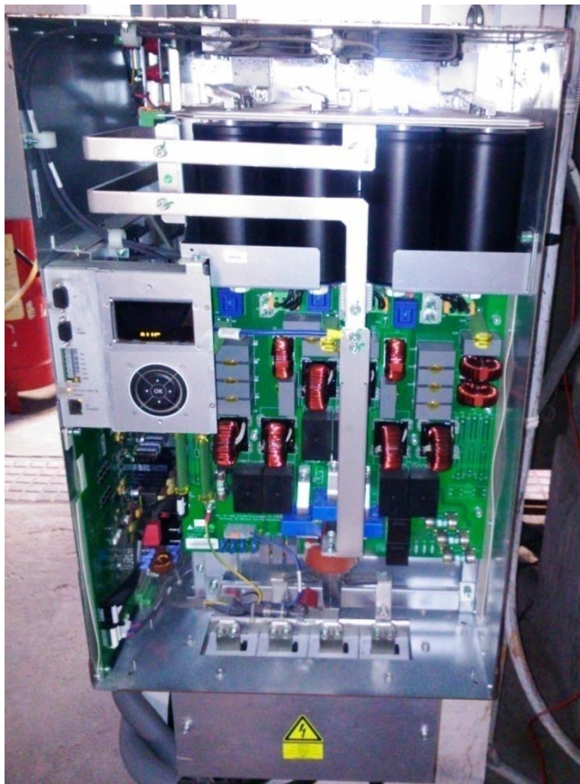
Installed Harmonic Filter at the Facility
