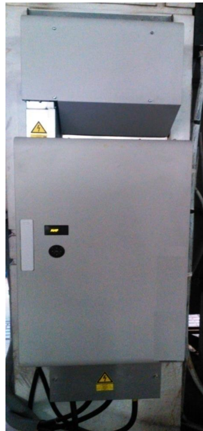
Installed Harmonic Filter at the Facility
